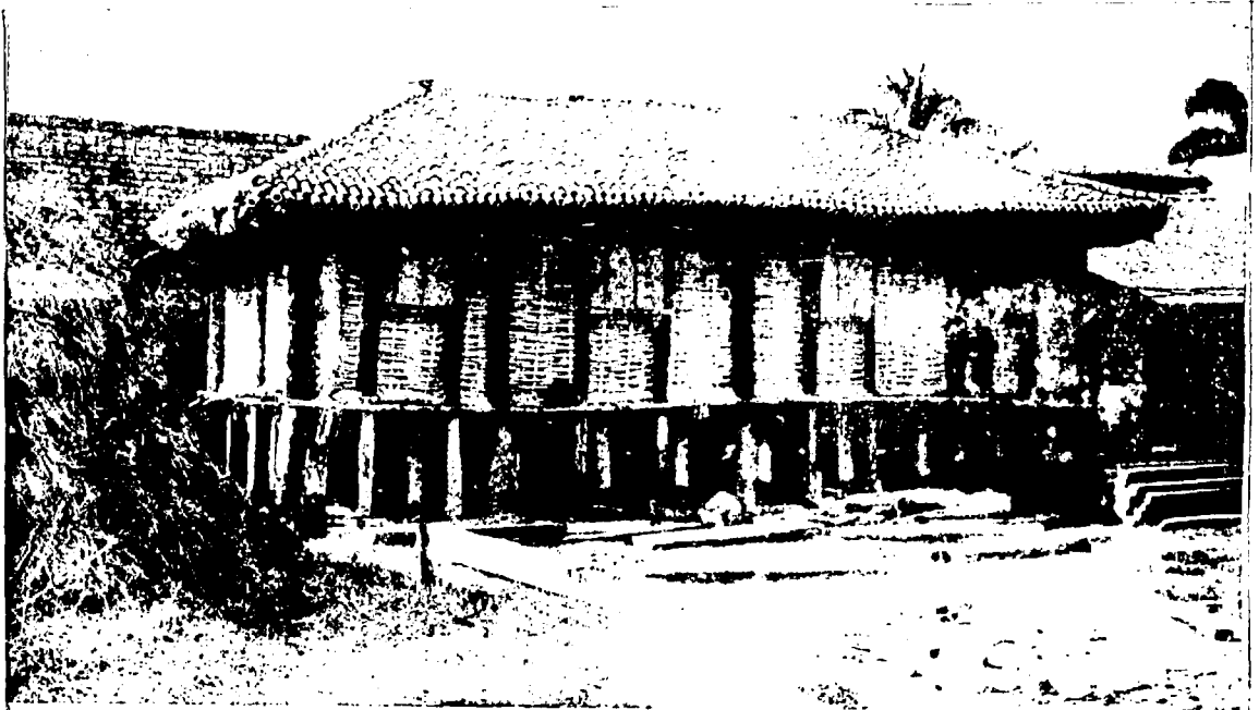
Fig. 1. A 'bukhari' under construction and almost ready for use. The walls of bamboo wattle, and the floor have not yet been plastered with mud.
