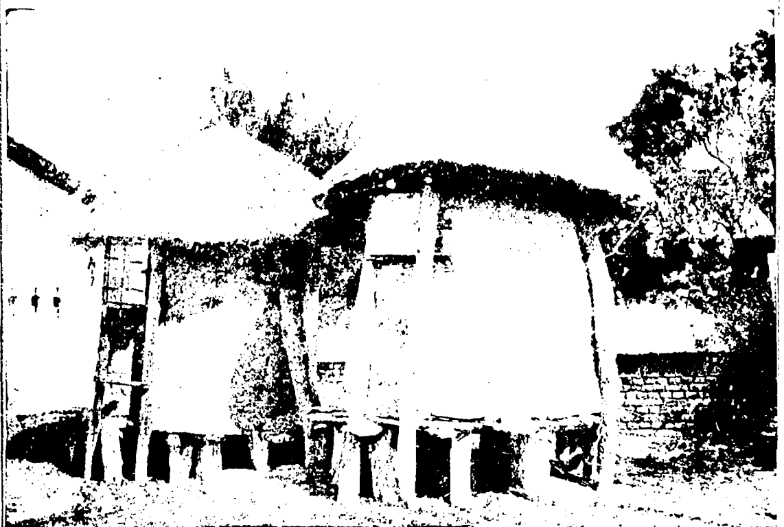
Fig. 2. Two 'bukharis' of a type common in Bihar for storage of grain.
