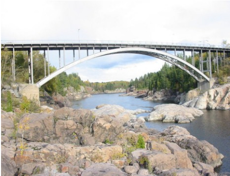
Fig. 1.3 Arvida Aluminium Bridge, Canada (Aluminum company of Canada Ltd, 1940)
