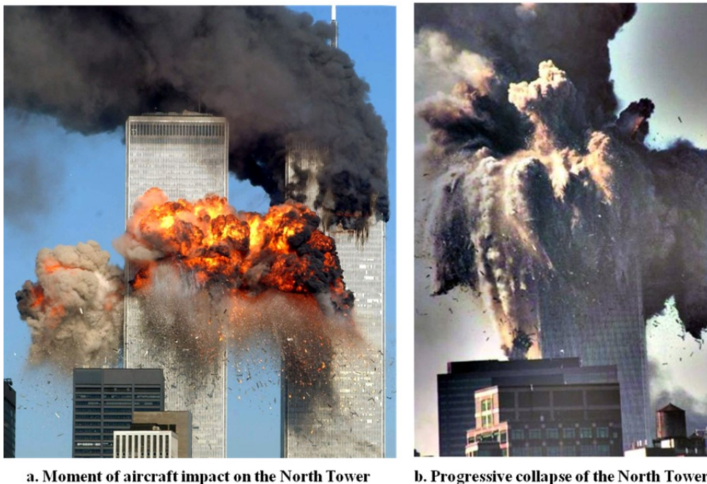
Figure 1-4: Collapse of the WTC Twin Towers
