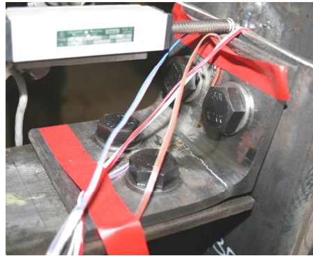
(a) Typical low-cycle fatigue fracture in top angle (Specimen T6.3-A8-d40-Y)
