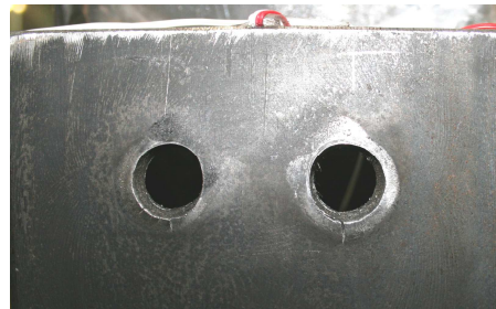
(b) Fatigue damage around bolt holes in reverse channel component (Specimen T6.3-A8-d40-Y)
