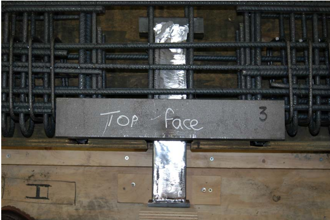
Figure 6: SPT2-3 detail with main reinforcement prior to casting
