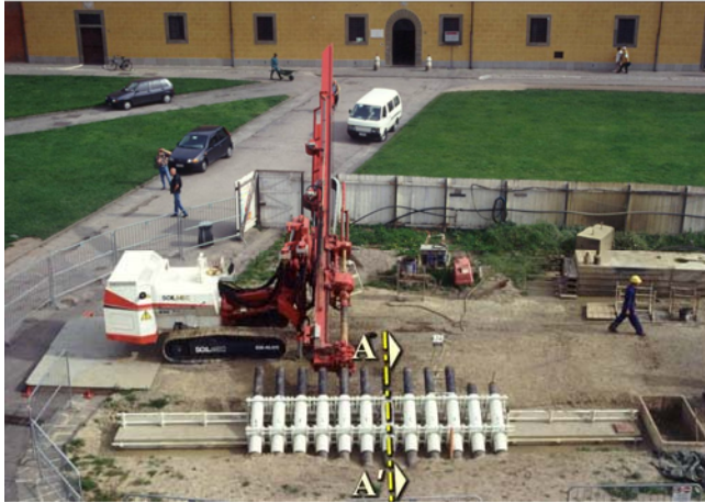
Figure 9. Holes for preliminary underexcavation.
