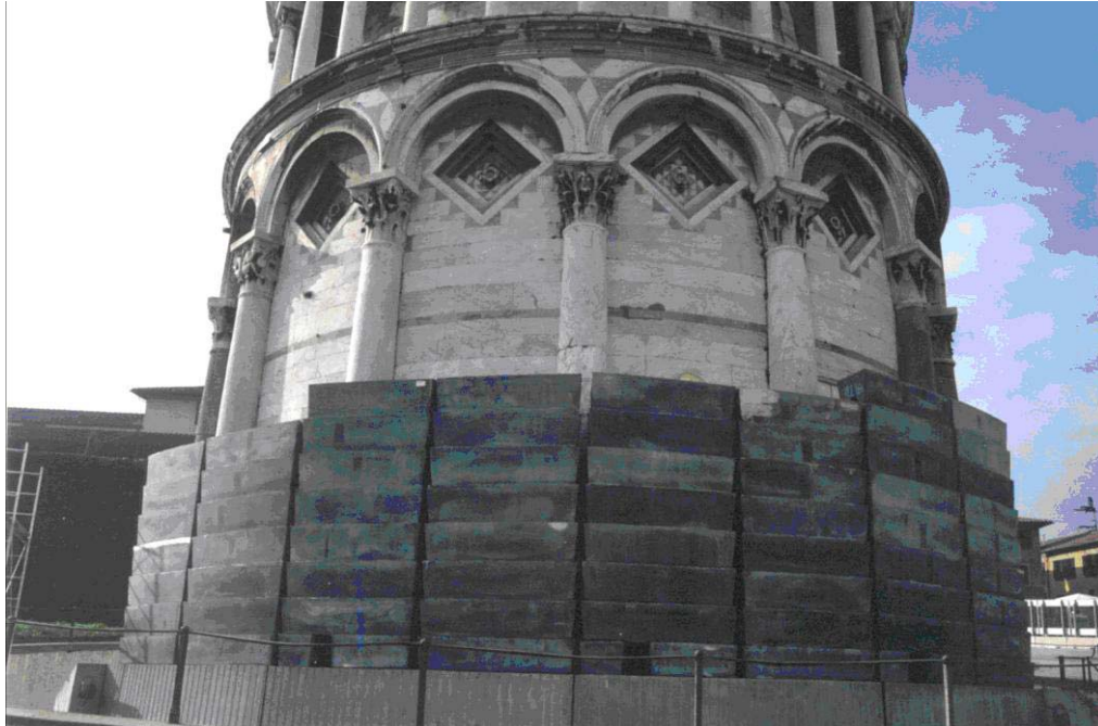
Figure 7. Lead counterweight on the North Side.
