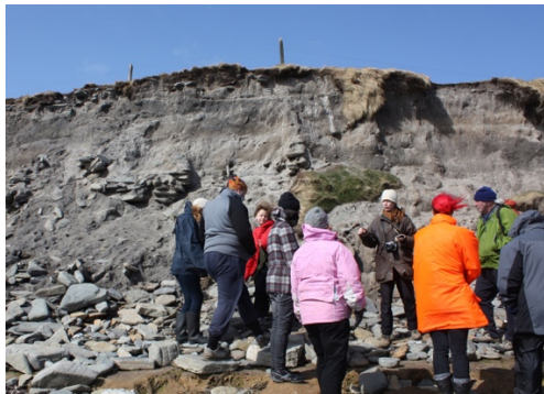
Figure 1: A ShoreUPDATE training event with SCHARP Project Manager, Joanna Hambly. Note the eroding structures in the coastal dune behind the group.
