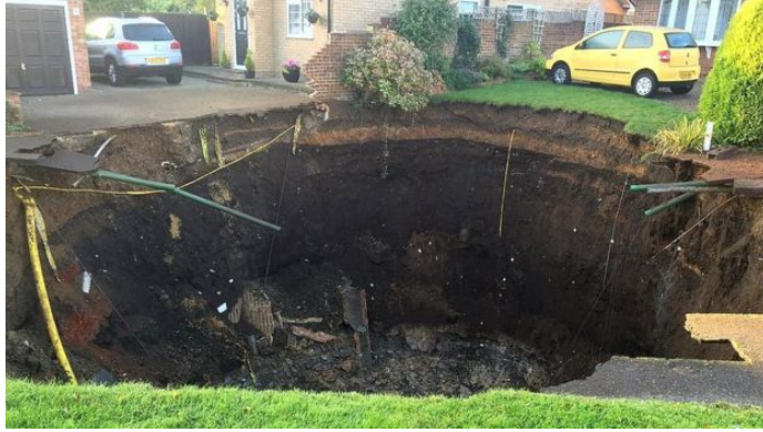
Figure 1.3: Large sinkhole formed in residential area due to underground soil erosion. Image courtesy of Hertfordshire Fire and Rescue Service 2015.
