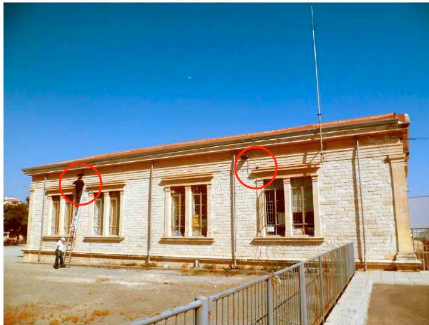
Fig. (24). Position of the 2 accelerometers at one side of the building.
