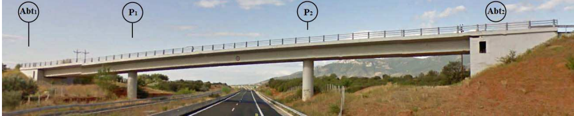
Fig. 2 Overpass T7, Egnatia Motorway, N. Greece (Google Earth 2011)
