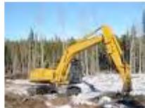
The Ground Prep Workers
