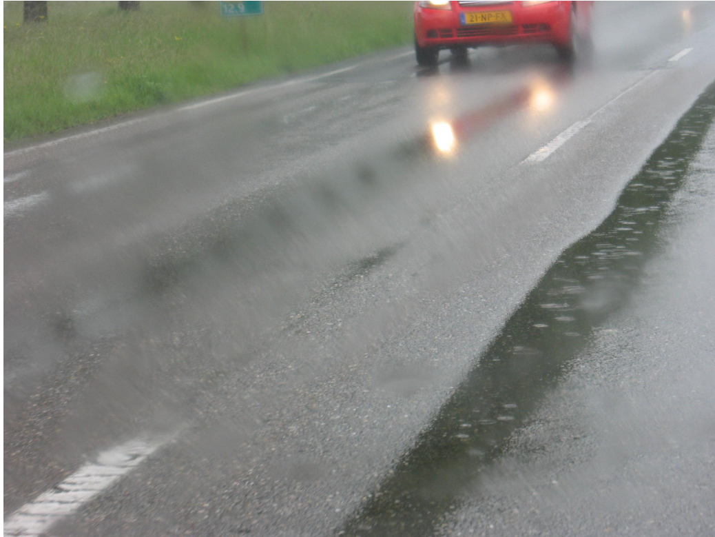
Figure 1.5: Hydroplaning problems in road pavements [Google Images]
