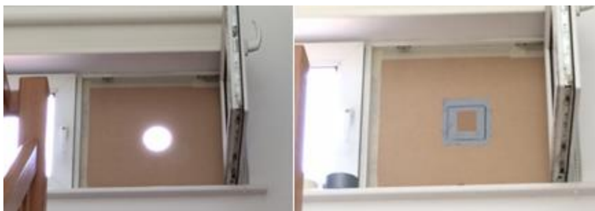
Figure 17: Setup of the known opening in house No. 8
