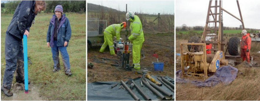
Fig. 4 Dipwells can be manually installed ( left ), deeper dipwells and piezometers can be installed into more competent material using portable hand-powered drills ( middle ), and larger percussion drills are used to install deeper boreholes and piezometers into bedrock
