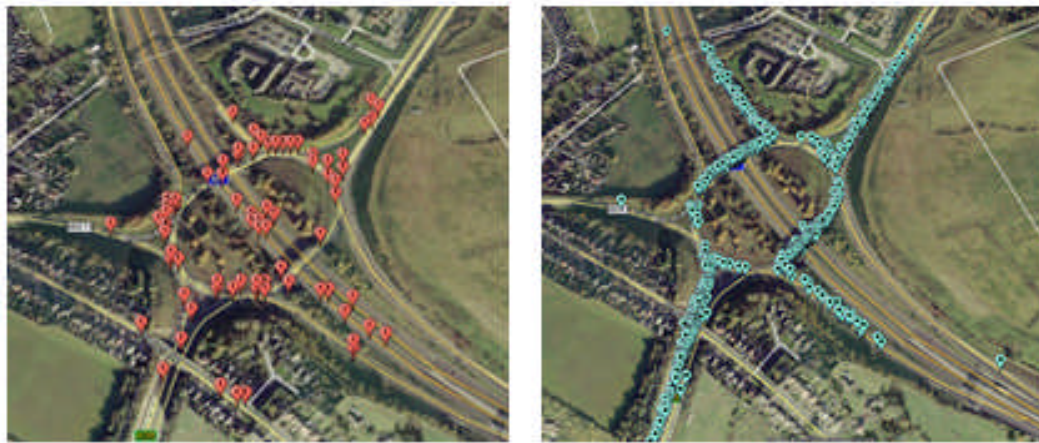
Figure 1-1 Grade-Separated Roundabout (J28 on the M1) with Accident and HBI Positions Geometric design of roundabouts is a sensitive case, as any sudden change in geometric design leads the roundabouts to be less safe as stated by Kennedy (2007). Truck rollover accidents are common at roundabouts (Kemp et al., 1987). Trucks overturn at roundabouts because of extreme speed or hard braking, while they are on adverse super elevation, as stated by Kennedy (2007). In addition, Arndt (1991) (cited in Kennedy, 2007) states that roundabouts with high inscribed circle diameter (ICD), with high speed, and when there is a high cross-fall at the circulatory lanes, leads trucks to be unbalanced. Weber et al. (2009) in a study for accommodating small and large trucks at roundabouts stated that issues with trucks at roundabouts mainly include accommodating trucks within the available geometry. This indicates that geometric design of the roundabout can highly influence truck drivers and may lead them to record HBIs and in such cases roundabouts become less safe for trucks if there were any sudden changes in its geometry. Moreover previous studies (illustrated in Chapter Two, Section 2.3) identified the influence of traffic and geometric variables on total accidents at roundabouts, and they found significant results regarding these influence. Therefore in this study, geometric and traffic variables (AADT, and percentage of truck traffic) were selected to identify their influence on total and truck accidents and on truck HBIs. This will leads examine if truck HBIs at roundabouts are influenced by similar variables that affected total and truck accidents.
