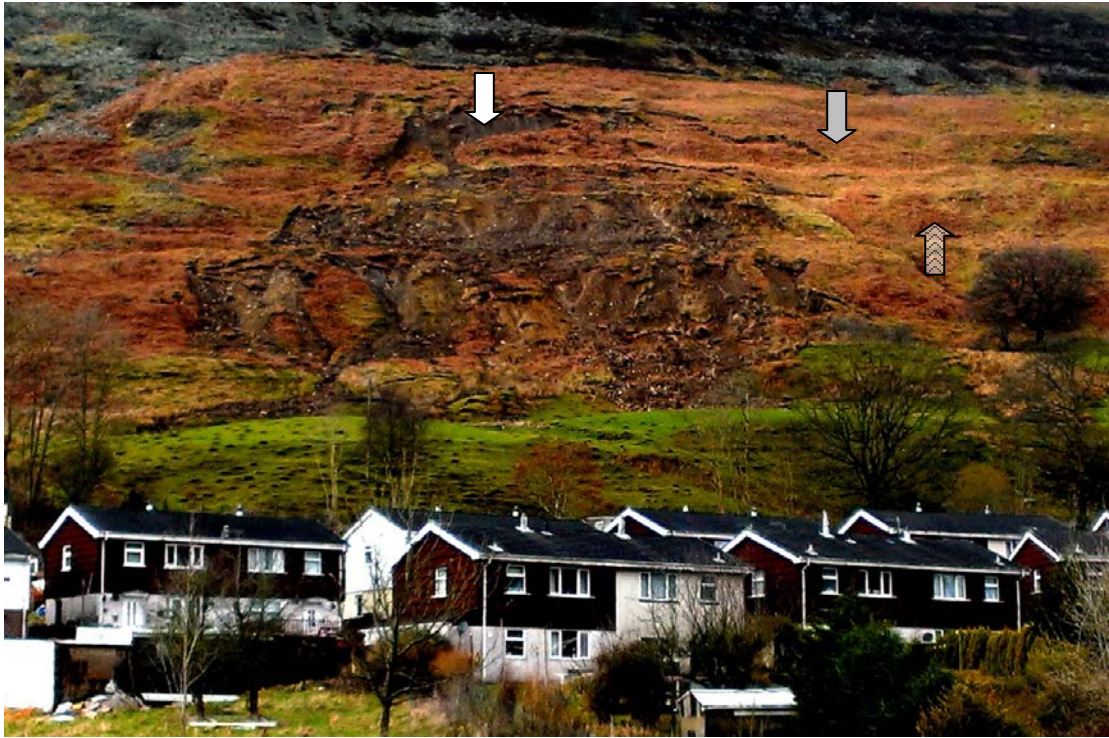
Figure 17 Photo of landslide-affected slope at Glan Ebbw taken 4 March 2016. Photo colour and contrast has been enhanced for clarity. Note the now well-developed main back scarp on the southern side of the crown (white arrow), crown cracks on the northern side (grey arrow, right side), and compression and bulging of topsoil at the toe of the upper-slope rotation (zig zag arrow, middle right). This feature is arguably present, though less well developed, in the earlier 23 December 2015 photo (Figure 1) indicating retrogressive movement. The upper row of houses is located along Glan Ebbw Terrace.
