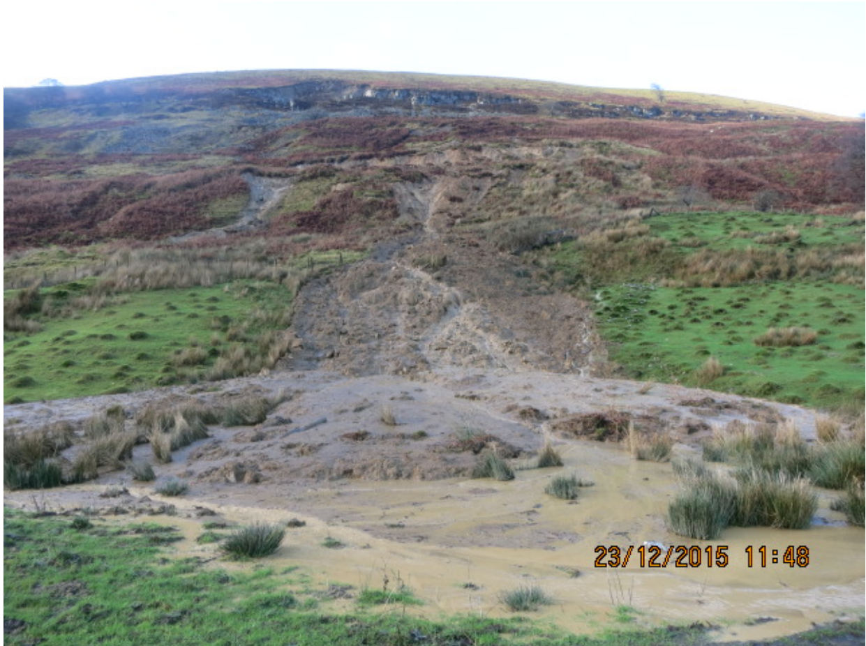
Figure 1 Photograph of landslide-affected slope taken on 23 December 2015, shortly after the initial movement took place. Note the accumulation of saturated landslide debris forming debris cones (wet clayey sand) over the flat area, which is the toe of an ancient landslide. Note how the alluvial fan is prograding out to the east, blocking the field drains and diverting sediment-laden water across the path and towards the houses below. (Photo Courtesy of BGCBC).
