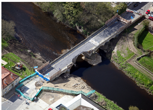
Plate 3 Aerial view of the flood damaged A659 road bridge in Tadcaster, Yorkshire. Photo: Neil Mitchell, Shutterstock.
