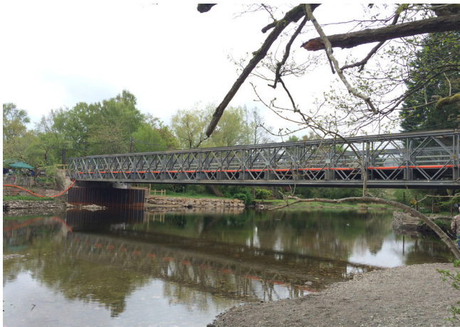
Plate 7 Temporary replacement for the collapsed Pooley Bridge, Cumbria. Photo: Katie Muchan, CEH.
