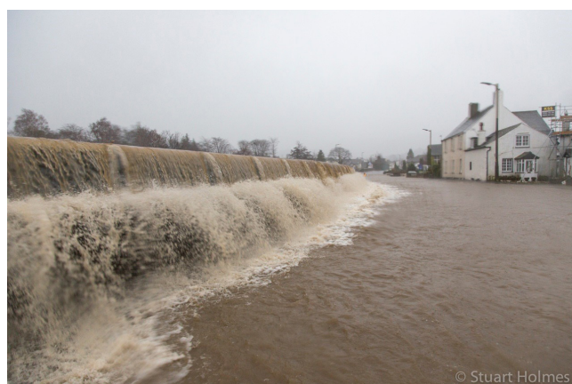
Plate 4 Keswick's glass topped flood defences before (above) and during overtopping (below).
