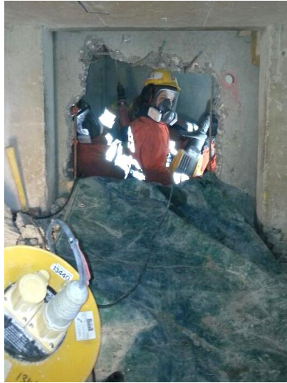
Figure 58 - Tool usage upside down in confined space
