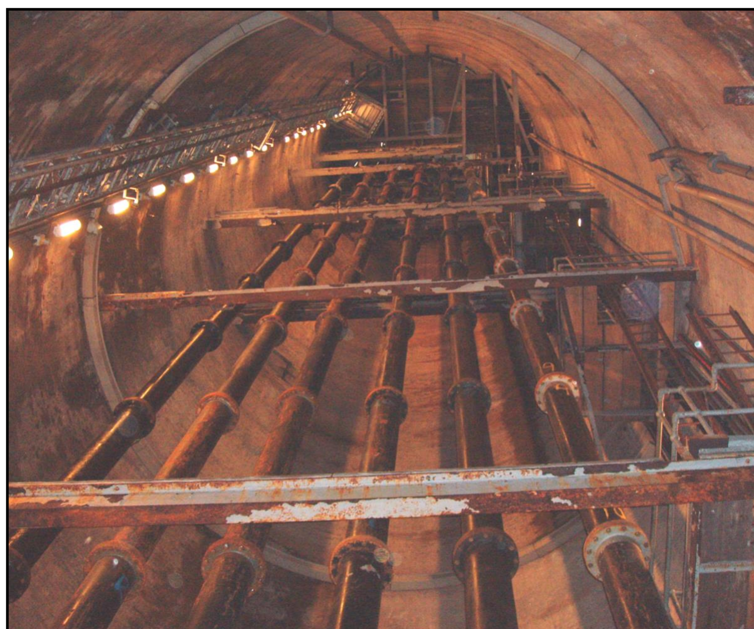
Fig. 2. Looking upwards in the pumping station
