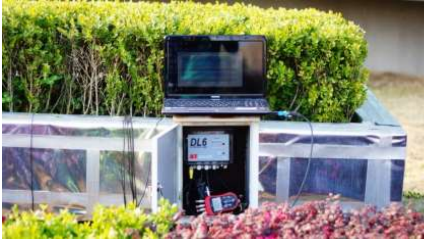
Figure 5-3: Thermal and moisture data logging facility installed at green roof test cell
