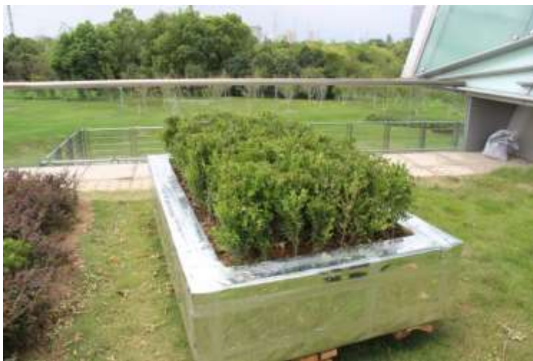
Figure 5-2: Completed test cell installation at CSET rooftop.
