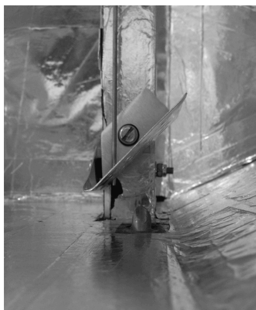
Figure 33 - A detail view of the pitot probe installed and projecting through the target.
