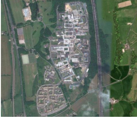
(a) Google Earth view of Lancaster University
