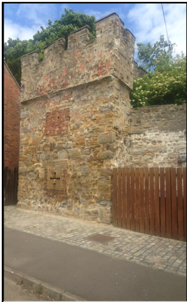
Figure 18. Silver Street Tower. Photograph taken from the western approach. Photographed by author.
