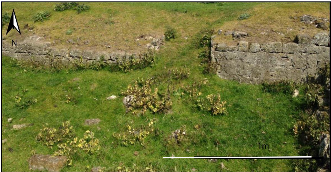
Figure 39. Photograph of the north wall of Feature D. In contrast with Feature F, this wall is mortared with evidence of a window or doorway. This feature is therefore a probable in situ wall. Photographed by author, 2015.
