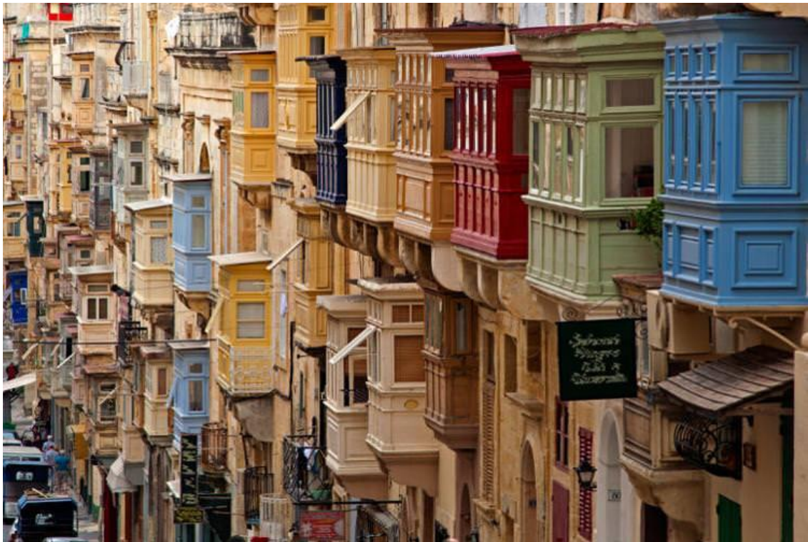
Figure 5.1: A multitude of balconies in Valletta showing the cramped housing environment
