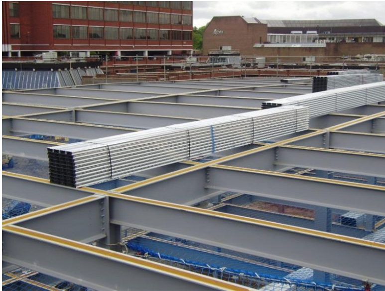
Figure 1 Composite beam grillage with profiled decking placed on the beams
