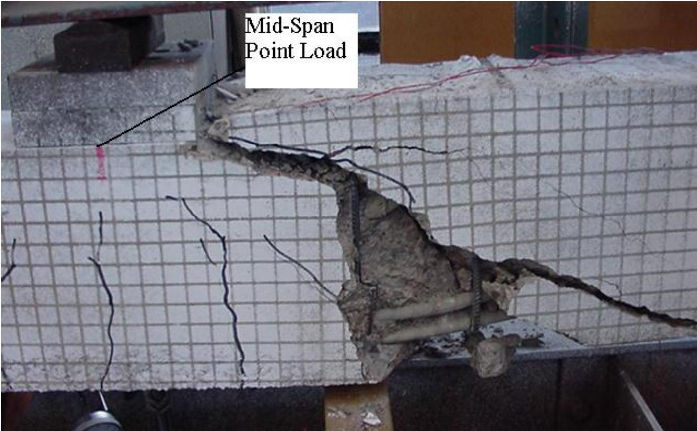
Figure 5: Flexure-shear failure of beam GcOO
