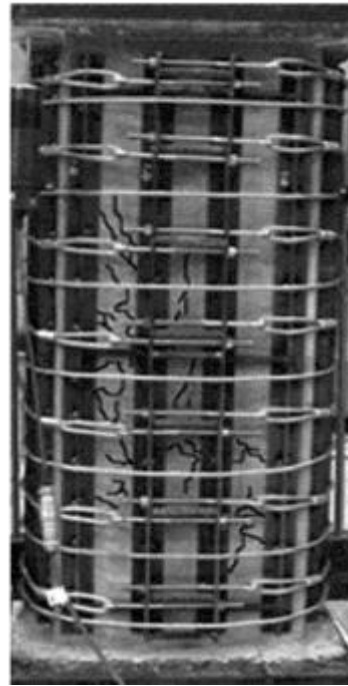
(b) Inclined cracks at ultimate strength
