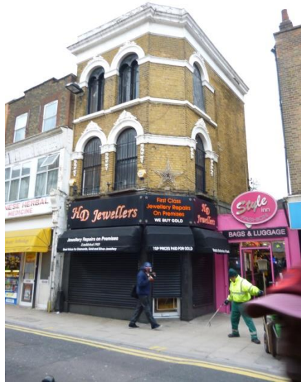
Figure 13.1. Shop front, Mare Street, surviving Victorian building with postwar infill
