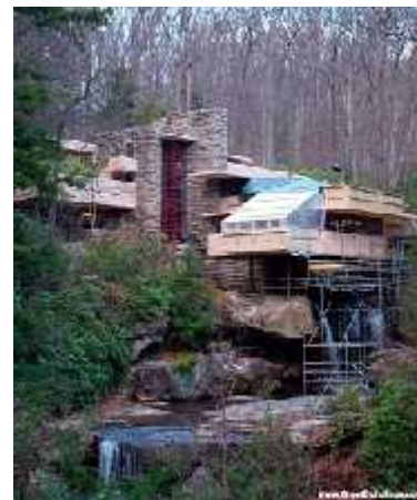
Gambar 2.6. falling water house
