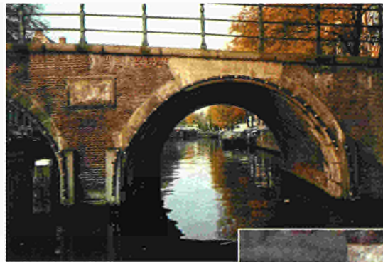
A bridge in Amsterdam, restored using data gathered by the Masonry Damage Diagnostic expert system and technical investigations, especially of the mortar.
