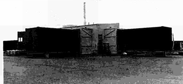
Fig.57: Waste Handling Facility.
