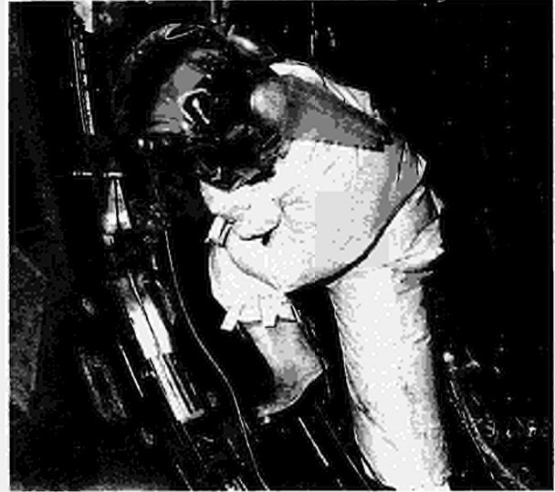
Fig.12: Removing redundant bosses welded to the vacuum vessel wall.
