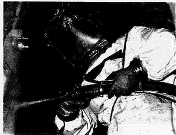
Fig.13: Cleaning the vacuum vessel walls.
