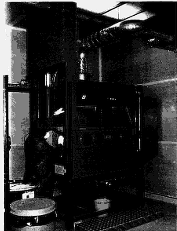
Fig.55: Grit blasting cubicle in Beryllium Handling Facility
