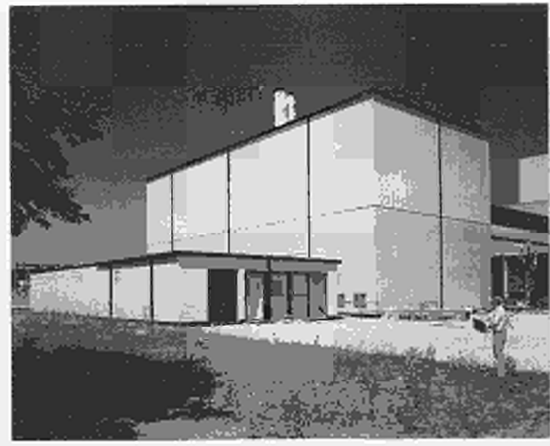
Fig.187: The AGHS Building in Summer 1990;
