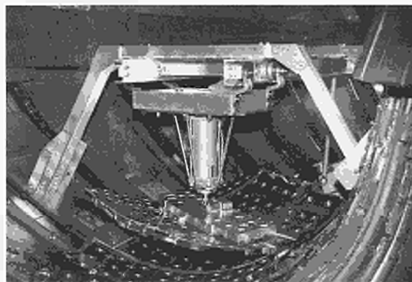
Fig.12 Continuous X-point dump plates during installation
