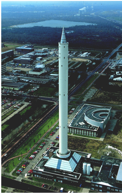
(a) Tower from the outside
