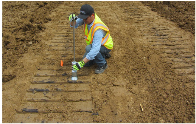
CEER in situ drive cylinder test at Linn County Project 4
