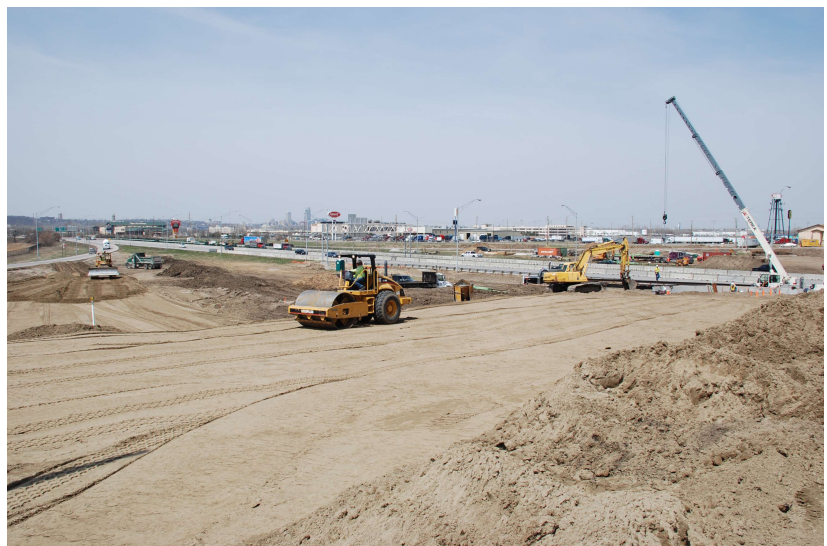
The location of the new 24th Street Bridge
