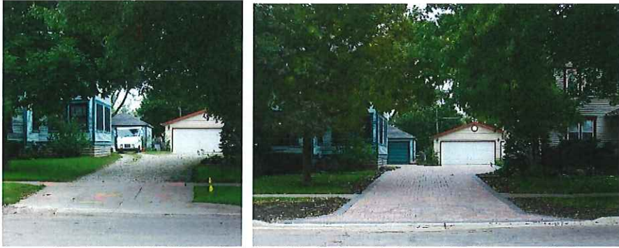
Jean Reavis and Vicki Bentley-Conditt's Before & After Joint Permeable Paver Driveway (1875 sq. ft.)
