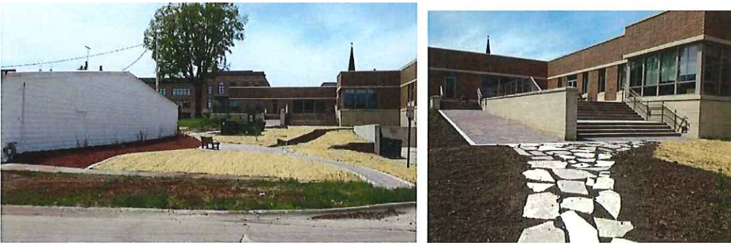
Drake Community Library After 1355 sq. ft. of Permeable Pavers on the South Side of Library
