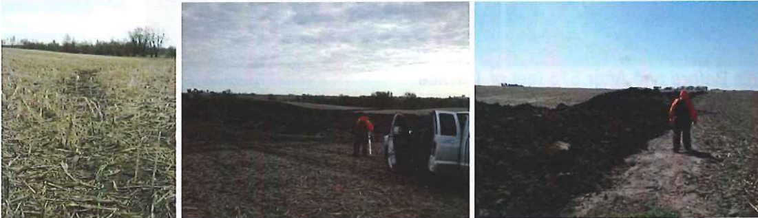
Caroldon's Before and After (North 2 Basins) and During Construction 2 South Basins
