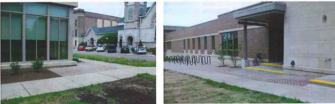
Drake Community Library After 579 sq. ft. of Permeable Pavers added on North Side of Library
