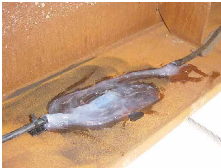
Figure 4.13. Completed splice after silicone protection has been applied
