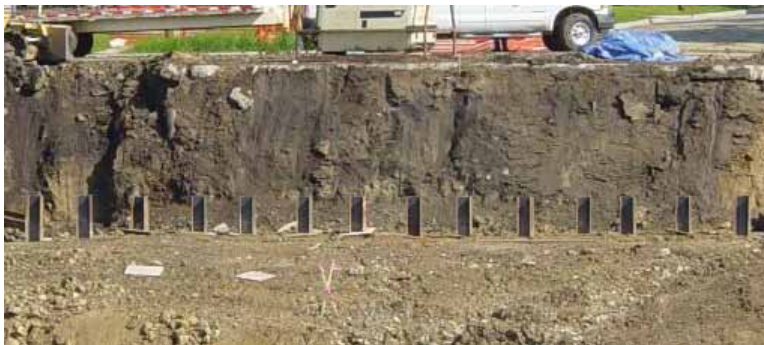
Figure 3.9. Piles at south abutment before abutment concrete was placed
