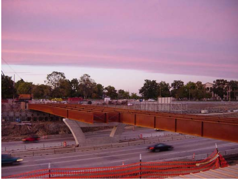
Figure 3.21. Girders installed after the second night of girder setting operations
