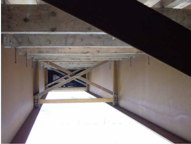
Figure 3.24. Intermediate cross-frames and deck formwork stringers
