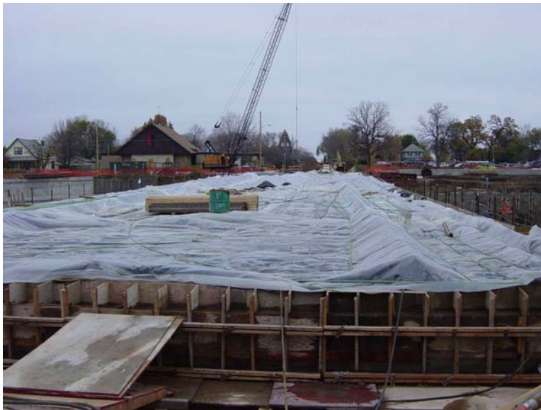
Figure 3.25. Bridge deck covered after concrete placement
