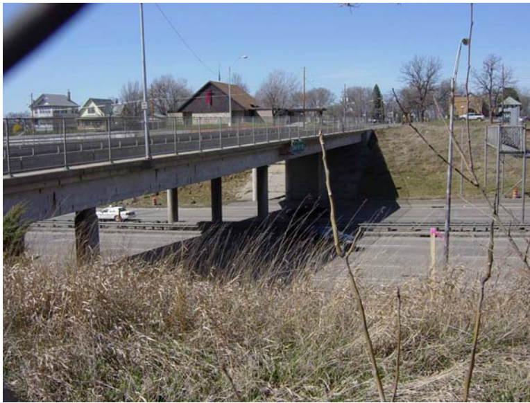
Figure 3.7. Original E. 12th St. Bridge
