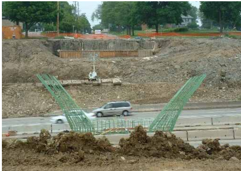
Figure 3.11. Reinforcing steel for the center pier
