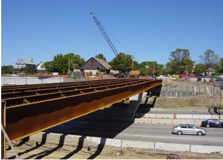
a. Side view of bridge
