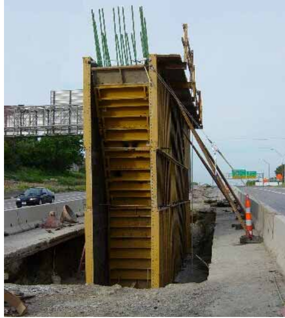
Figure 3.14. Center pier formwork after assembly and placement
