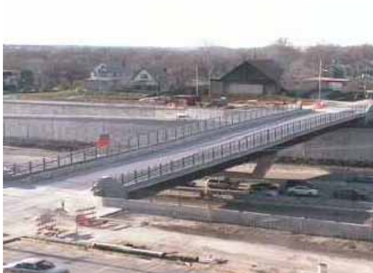
Figure 3.27. Completed bridge open to traffic
