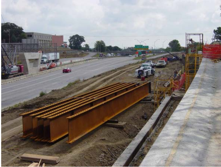
Figure 3.19. Stockpiled HPS girders located on the south side of I-235
