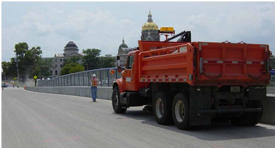
b. Load truck during run 2 of the controlled load test
