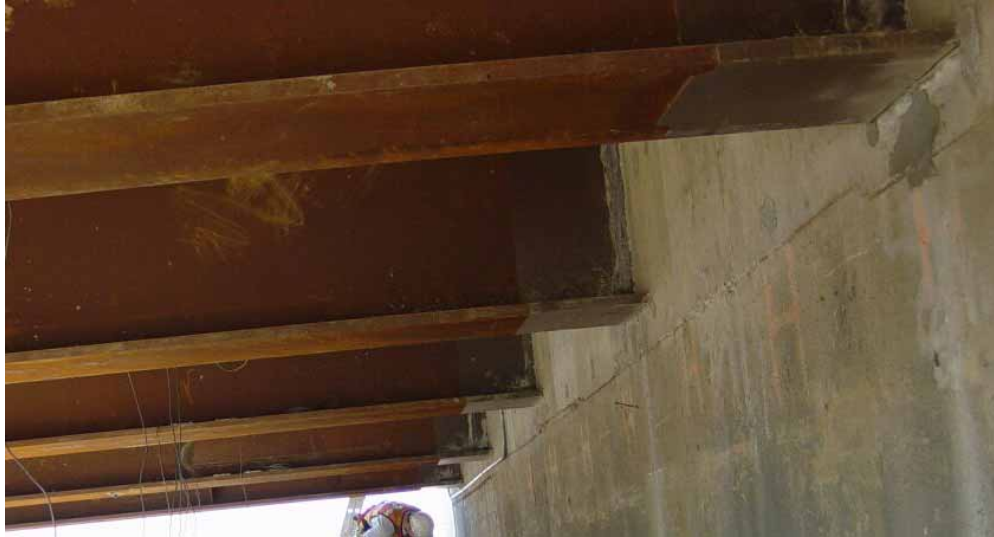
Figure 3.2. Typical girders and the north integral abutment
