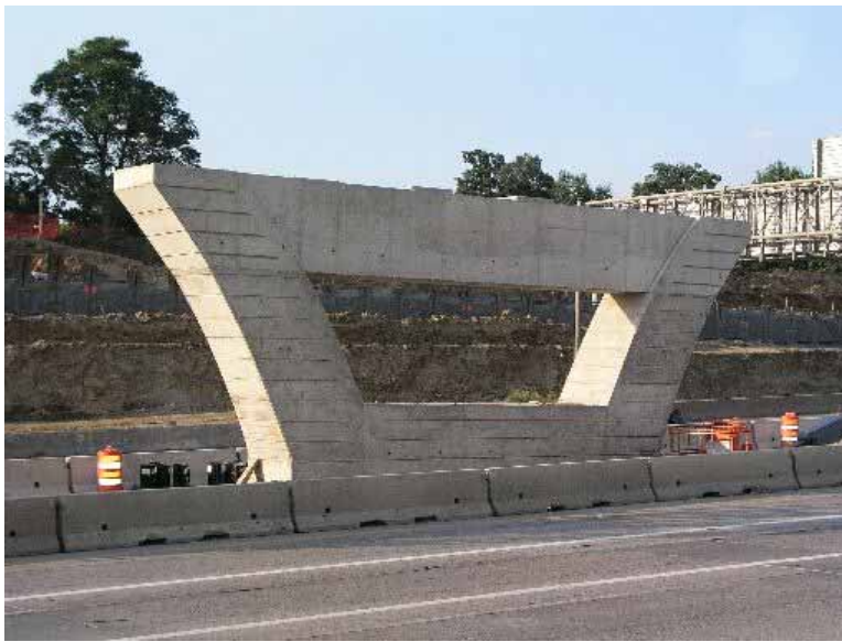
Figure 3.17. Completed center pier
