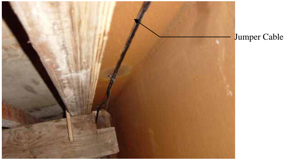
Figure 4.10. Jumper cable installed on top flange of girder
