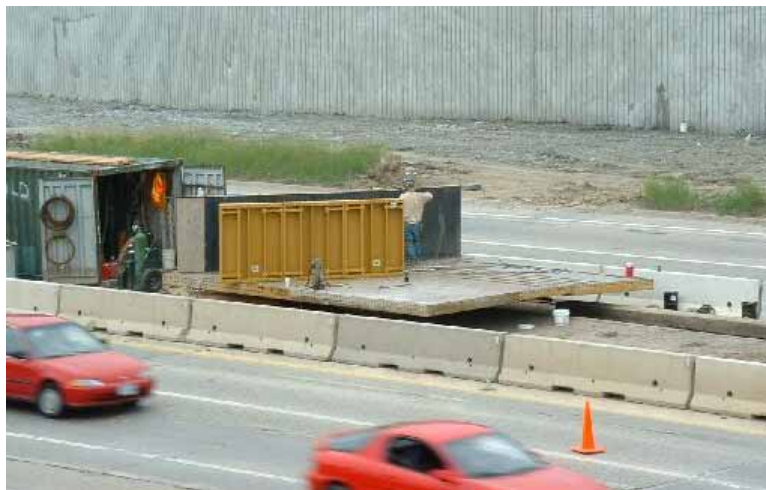
Figure 3.13. Formwork for the center pier during assembly
