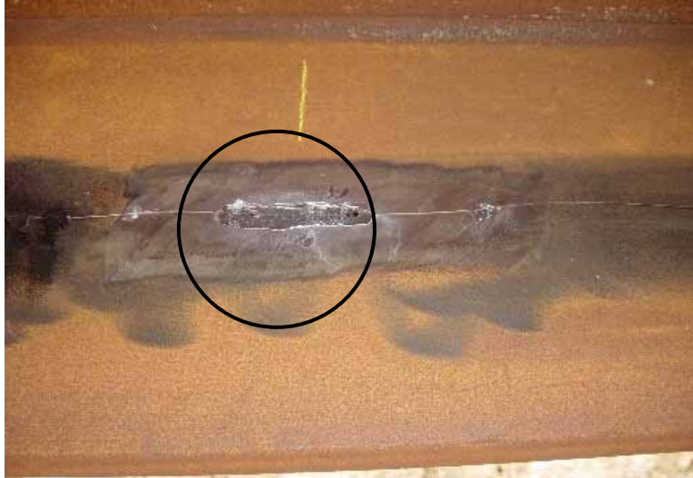
Figure 4.8. Single bare FBG sensor after installation
