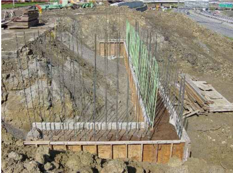
b. Top view of abutment
