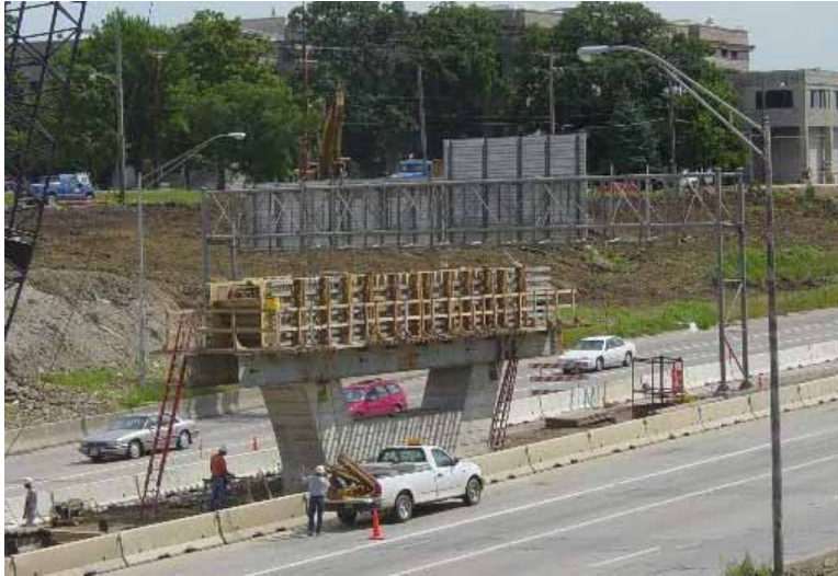
Figure 3.16. Formwork for the center pier cap being constructed
