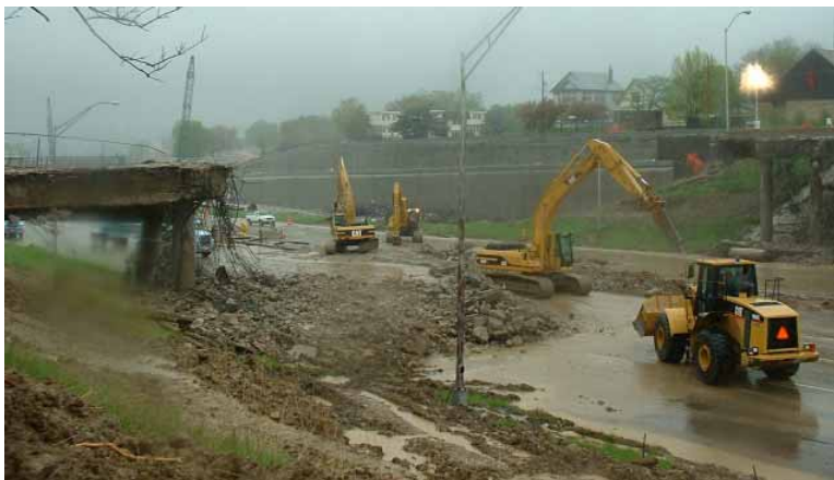
Figure 3.8. Demolition operations on Sunday, May 4, 2003
