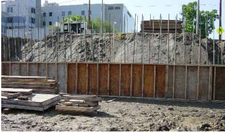
a. Front view of abutment
