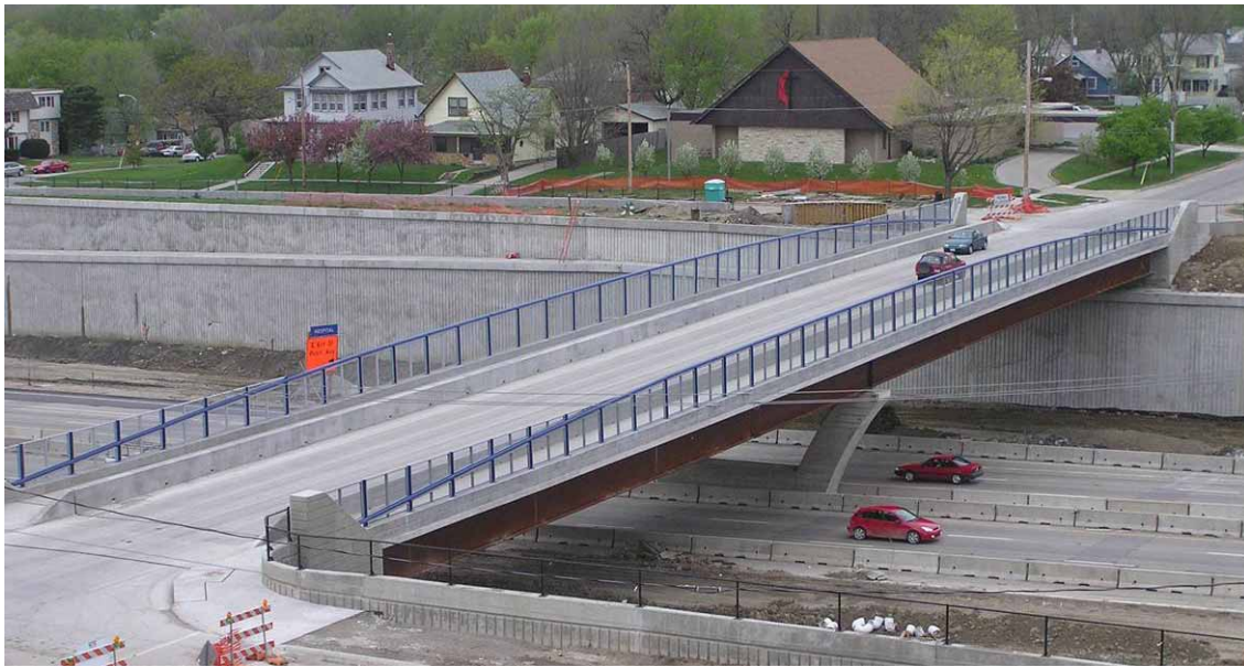
Figure 1.1. East 12th Street Bridge over I-235 in Des Moines, Iowa
