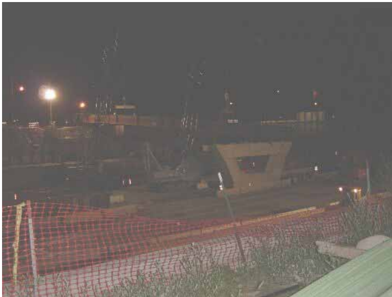
Figure 3.20. HPS girder being set during the first of three nighttime operations
