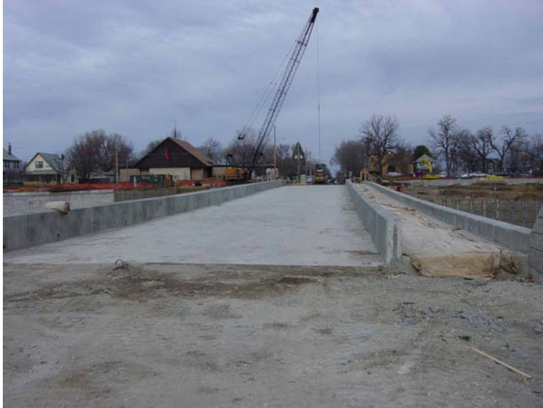
Figure 3.26. Bridge after slip forming of barriers
