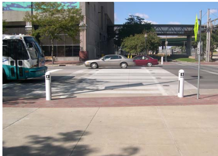
Figure 4. Crosswalk at ground level, looking northbound
