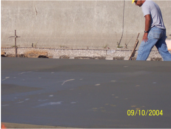
Figure C.5. Bleeding on the Slab Surface, Kansas Shadow Project
