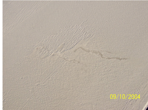
Figure C.5. Bleeding on the Slab Surface, Kansas Shadow Project
