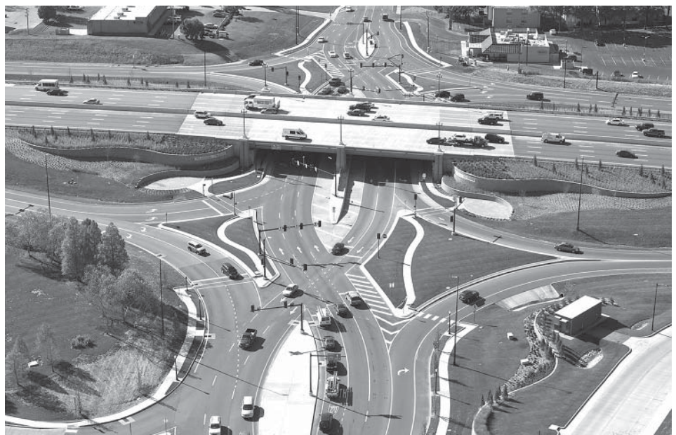
Aerial view of a diverging diamond interchange at I-270 and Dorsett Road in Springfield, Missouri
