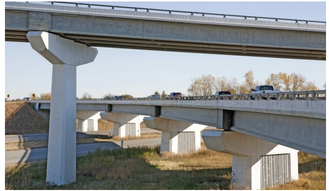
Figure 3-8. 3D engineered models can assist designers with visualizing important staging concerns in complicated projects.
