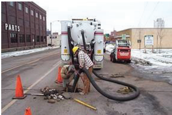
Figure 2-25. Hydro excavation operation to locate underground utilities.
