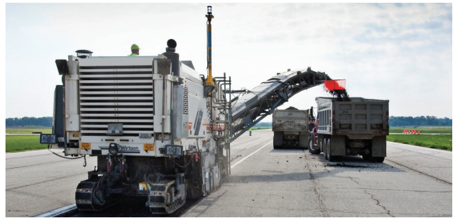
Figure 4-9. Stringless technology mounted on a milling machine.
