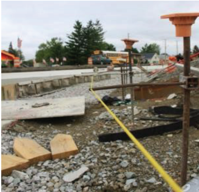
Figure 4-12. Traditional stringline near a curve.
