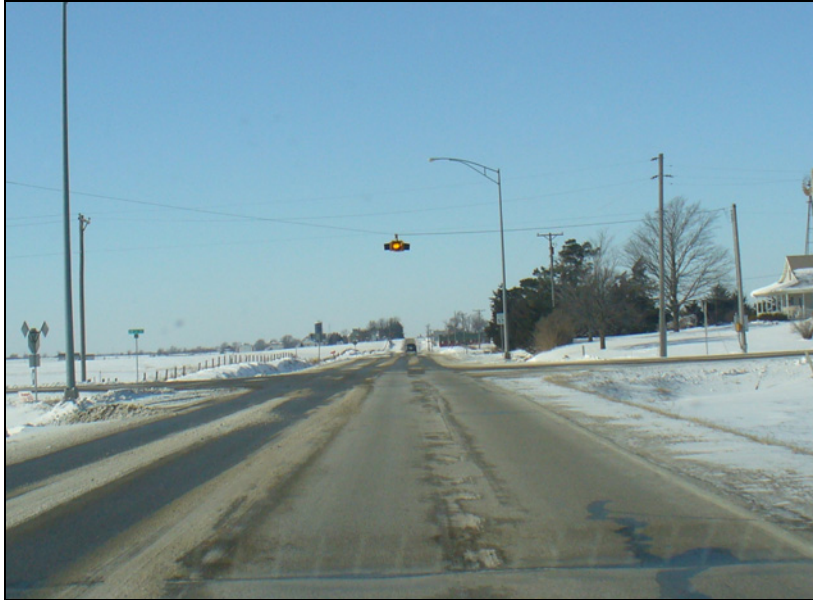
Figure 8. Use of overhead flashing yellow beacon at stop/through intersections (Image source: Neal Hawkins)
