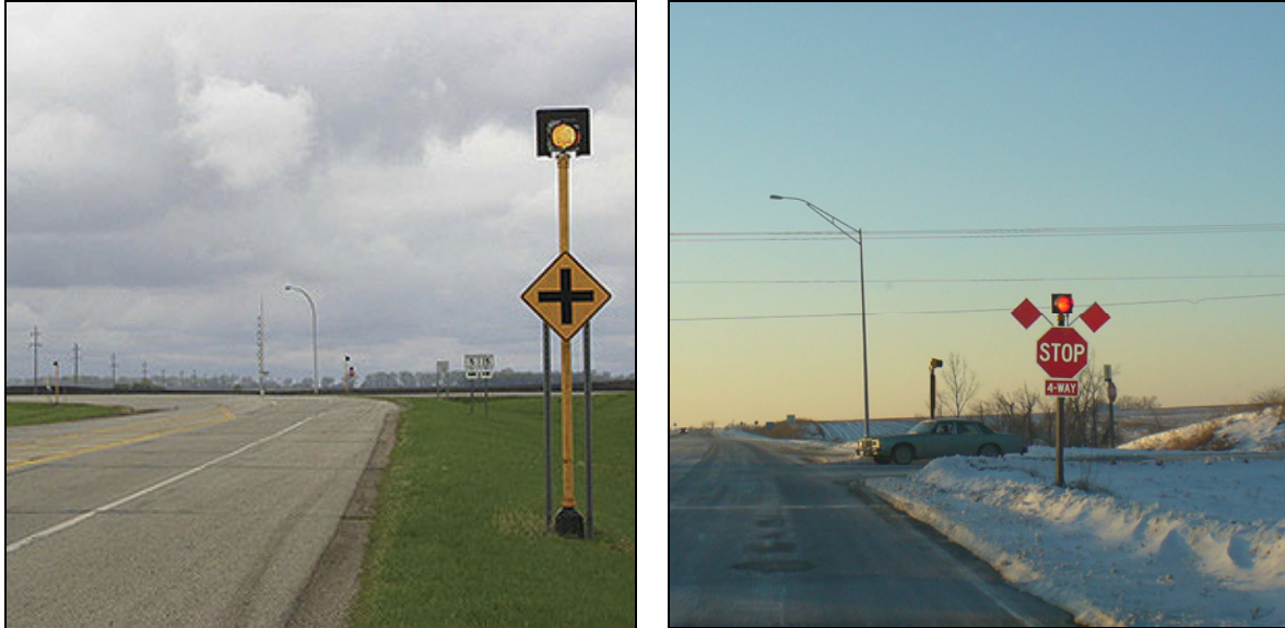
Figure 4. The Minnesota DOT's sign-mounted beacons used to replace overhead flashing beacons (Right image source: Mn/DOT from Amparano and Morena, 2006, Left image source: CTRE)
