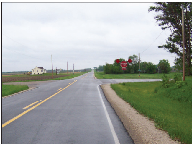
View of flags on Stop sign (photos courtesy of Bob Sperry)
