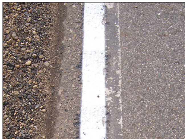
After milling (left) and with paint applied (right) (photos courtesy of Bob Sperry)
