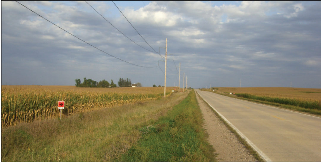
Poles moved back to ROW line (photo courtesy of Bob Sperry)
