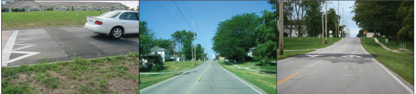
30 mph speed table used in the CTRE study for residential traffic calming (photos courtesy of Shauna Hallmark)
