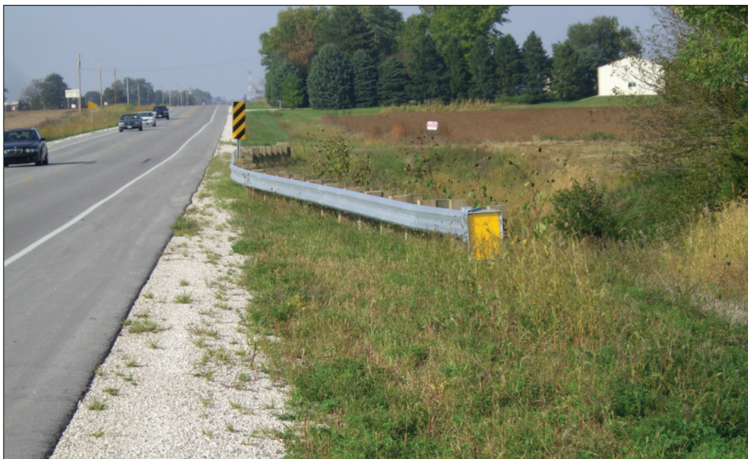
Guardrail provides protection from drop-off hazard (photo courtesy of Bob Sperry)
