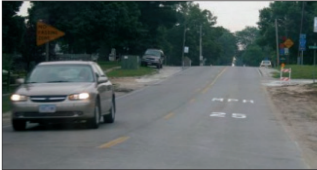
Speed limit pavement markings in Roland, IA (photo courtesy of Shauna Hallmark)
