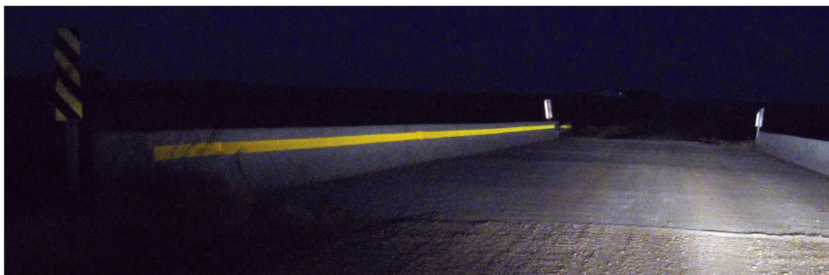
Reflective paint on guardrails (photos courtesy of EZ Liner Industries [top] and Bob Sperry [bottom])
