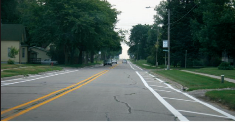
Shoulder marking completed (photo courtesy of Shauna Hallmark)
