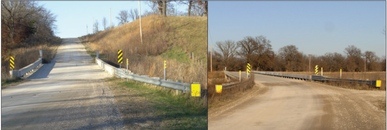
Approach guardrail on typical bridges (photos courtesy of Bob Sperry)
