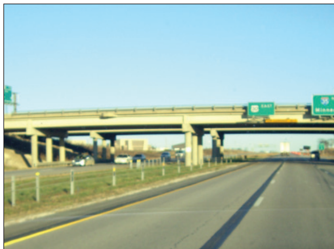
HTC protection of bridge pier (photo courtesy of Bob Sperry)
