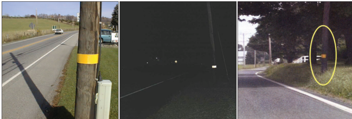
Simply adding a reflective tape to a pole or tree that cannot be removed may prevent a crash (photos courtesy of Jack Latterell, FHWA Office of Safety)
