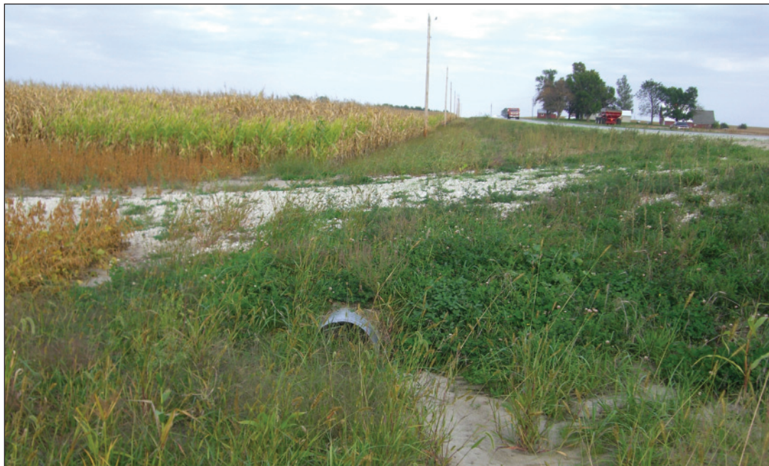
Additional culvert provided to flatten entrance slopes (photo courtesy of Bob Sperry)
