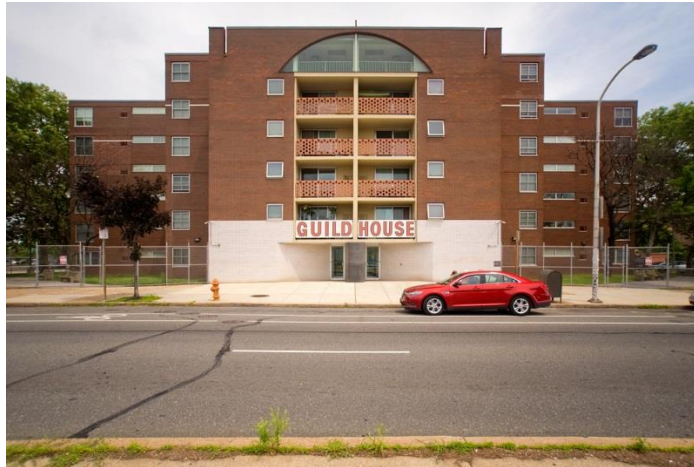
Fig. 8. Fachada principal Guild House (1963)
