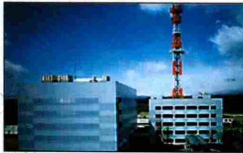
Fig. 3.17 Tohoku Electric Power Company, Japan.
