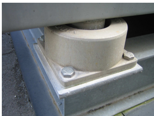
Figure – Vibration eliminator
