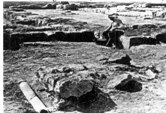
Figure 2.46: Clay drainpipe in Bathroom B and Lavatory A at the Palace of Lachish, looking northwest (Tufnell 1953: Pl. 23: 1)
