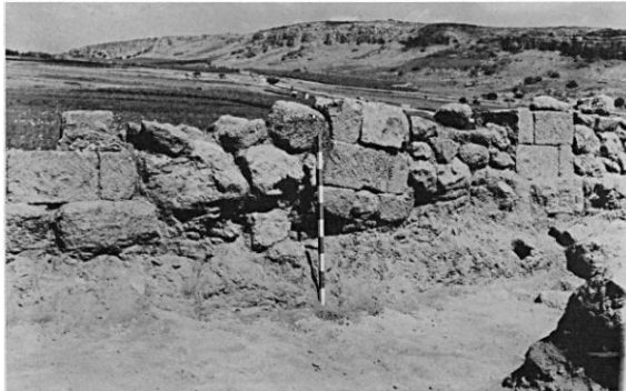
Figure 2.76: The inner casemate wall of Building 264 of Tell Mevorakh (Stern 1977: Fig. 6)
