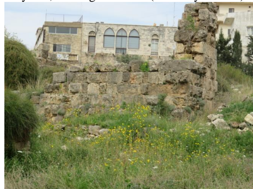
Figure 3.20: Tower no.5 of the Persian Complex at Byblos, looking northeast (Photo by Author)
