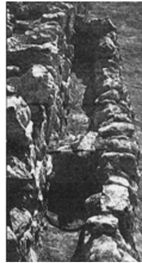
Figure 2.32: An enclosure along the northern wall of Hall 3001 (W2) of Citadel II Hazor (Yadin et al. 1958: Pl. XVI: 2)
