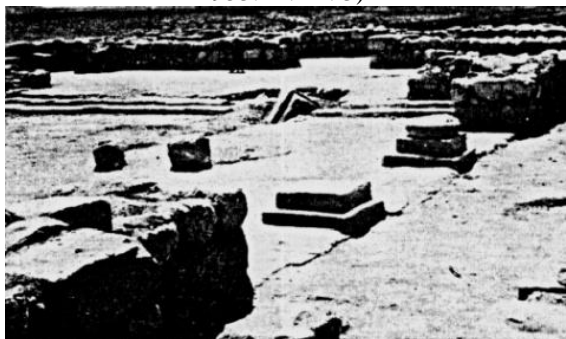
Figure 2.42: West and south porticoes of the Palace of Lachish with column basis in situ, looking southeast (Tufnell 1953: Pl. 22: 4)
