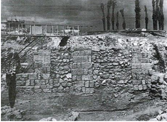
Figure 2.81: Wall from Building M of Jaffa showing the Phoenician technique “pier-and-rubble” (Kaplan and Ritter-Kaplan 1993a: 658)
