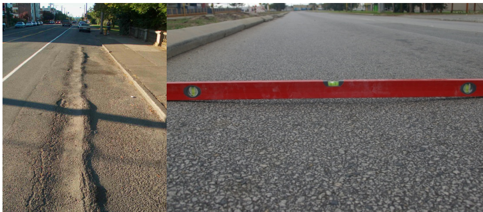
Figure 3.25 Rutting phenomena on surface layer.
