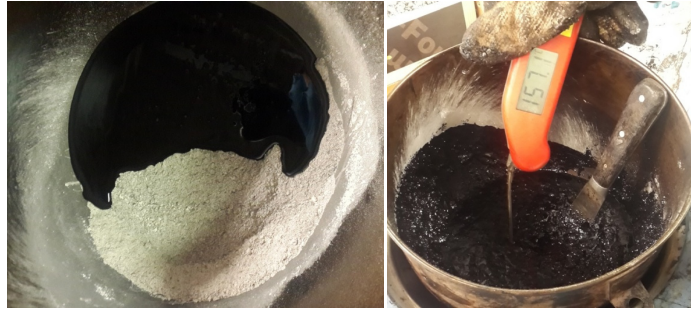
Figure 6.24 Mortar mixing process.
