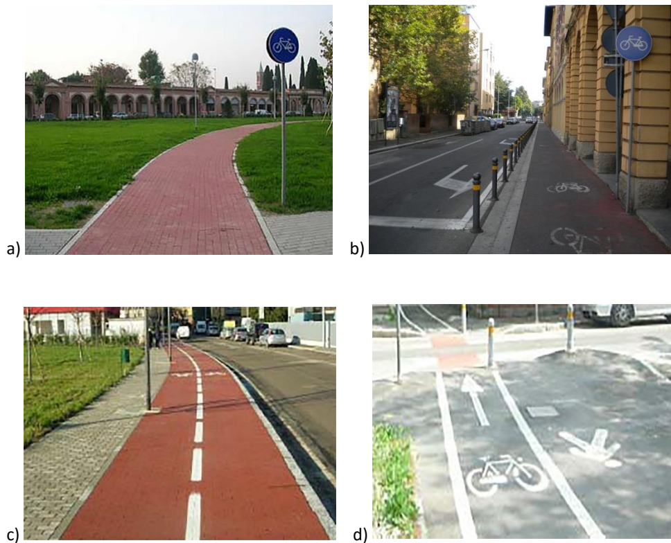
Figure 1: Some examples of the off-street facility typologies in Italy, as categorized in the Italian regulation: a) separated path non-adjoining the roadway; b) separated path, separation obtained by a non-continuous barrier; c) cycle track, obtained from the sidewalk, separating pedestrian and bicycle areas with different pavements; d) cycle track, obtained from the sidewalk, separating pedestrian and bicycle areas by painted markings.
