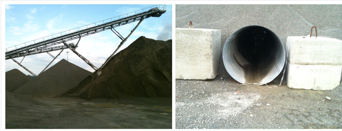
Fig. 5.4: disposition of stockpiles in plant and drainage pipes used to reduce the humidity of aggregates
